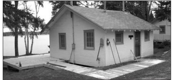
The new deck on cabin #1 wraps around with a level walkway connecting to the door. Landscaping was done to cut down the hill slightly in the front. Still needed are railings and to trim the rafters that overhang the deck.
