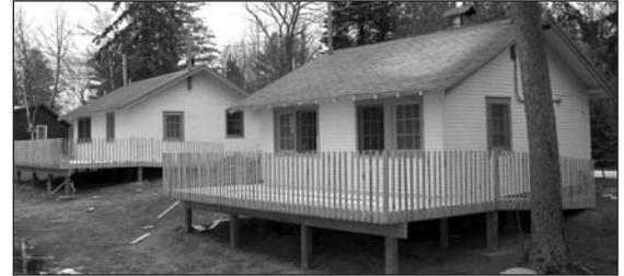
Cabin #2 and #3 decks almost complete. The last step is constructing the railing tops.
