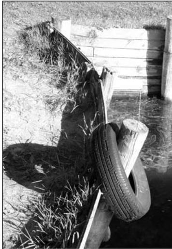
The harbor walls have been caving more each year. Anchor cables have slipped, poles are weakening and the original design and installation has not withstood the pressure.
