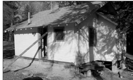
The first project this fall was to jack up #7. The cabin has been sinking a little each year, and this spring Mike noticed it was pinching off the water line. Time to git 'er done! The cabin was raised up about 18 inches. The deck will be reattached in the spring.
